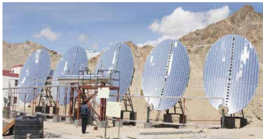
Picture 1: Scheffler dishes installed at Jawahar Navodaya Vidyalaya, Leh, Ladakh Source: Ladakh Renewable Energy Development Agency (LREDA)
